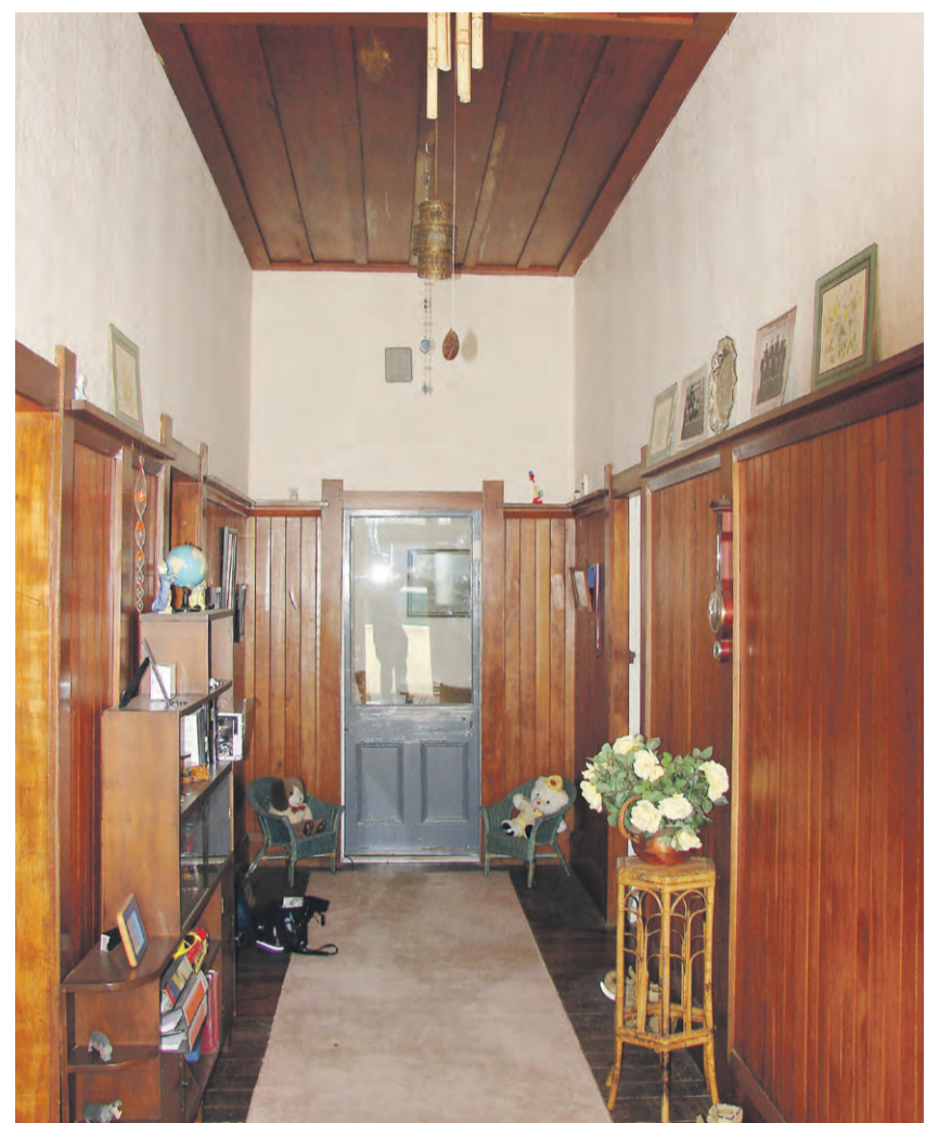
A hallway with character with rimu ceiling and rimu wall panelling
